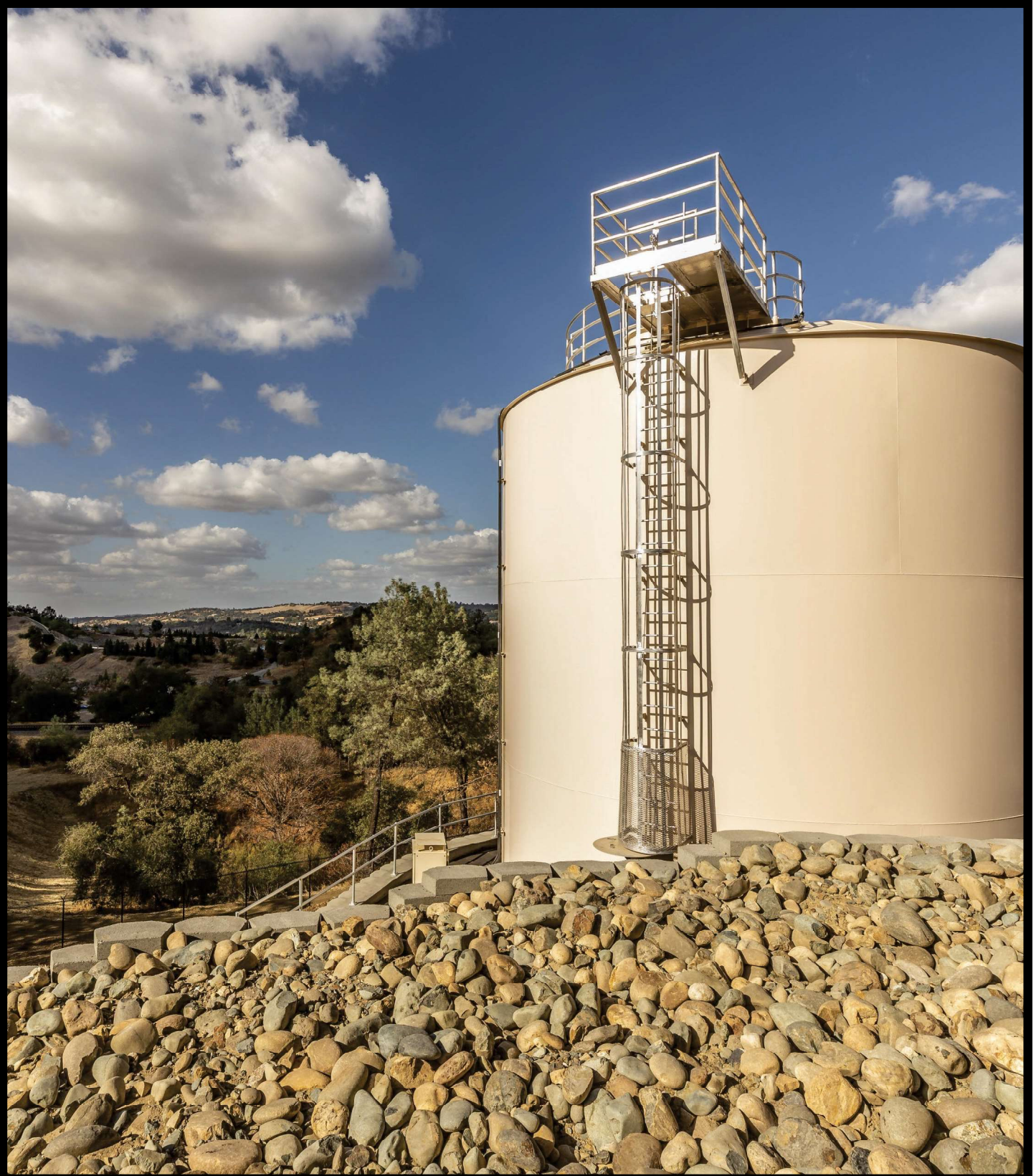
100,000 Gallon Standpipe, Foothill Raw Water Pipeline Project
