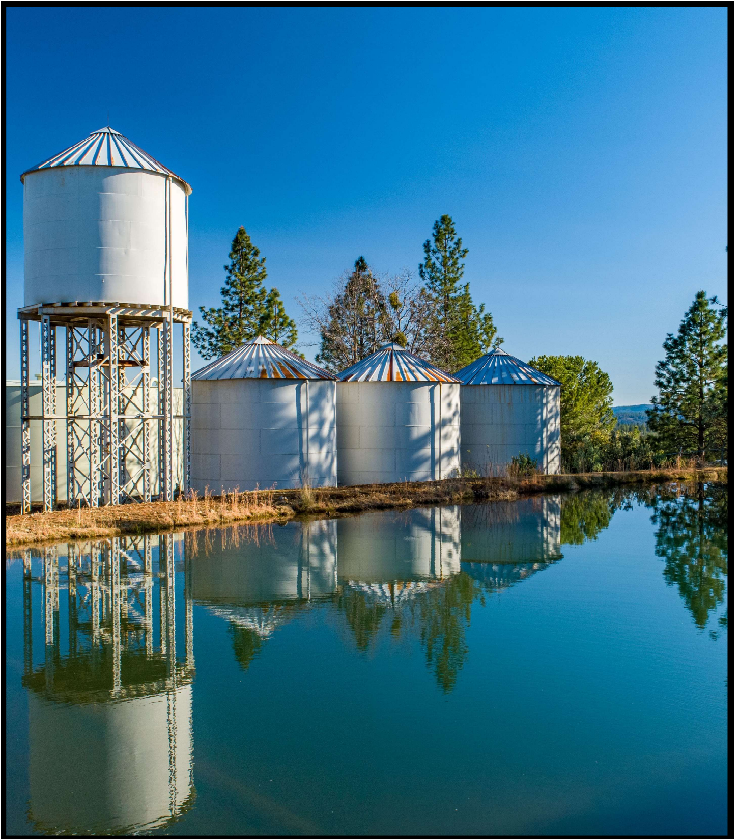
Water Storage Tanks and Reservoir, Weimar
