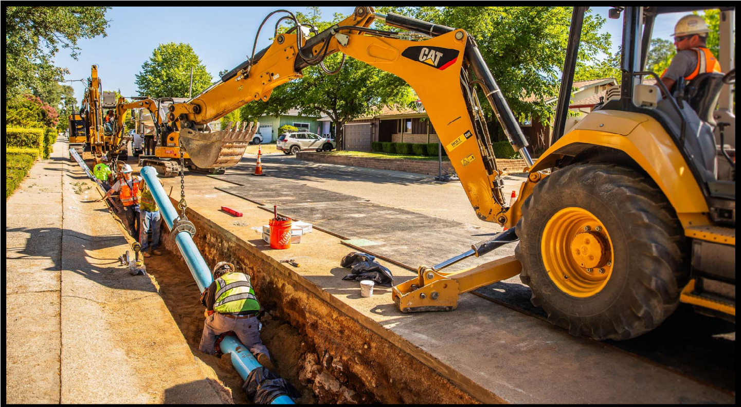
Ginger Drive Pipeline Replacement Project, Auburn
